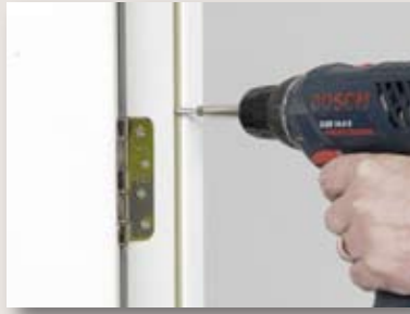
STEP 8: Screw through the lining into the wall where machined for the door stops, in recommended fixing positions to further strengthen the fitting of the doorset. (See image below)
