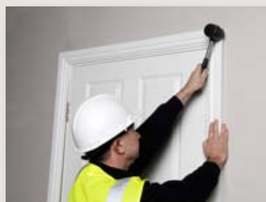
STEP 14: Add the final vertical piece of architrave, using a soft mallet if required. Make sure all is level. Repeat steps 11 to 15 on the reverse side of the door. The installation process is now complete.
