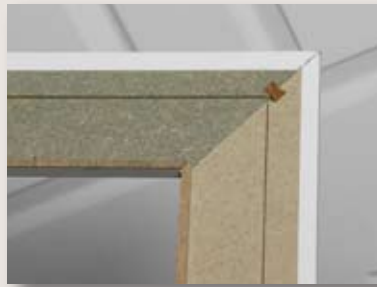
STEP 11: Using the Hoffmann Key provided assemble both pieces of the architrave together.
