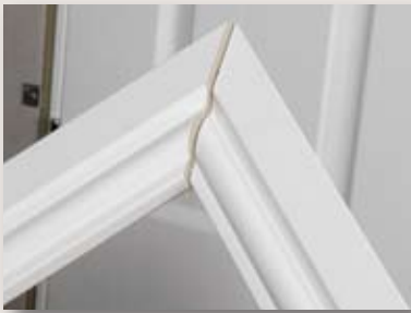
STEP 10: Take two pieces of the architrave, one edge and the top piece and offer them together.
