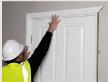
STEP 13: Press the two pieces of architrave in place, making sure that all areas are clicked into position and the corner joint is a tight fit.
