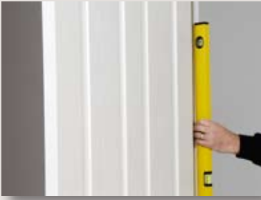
STEP 7: Make sure the door and the frame is plumb and square.
